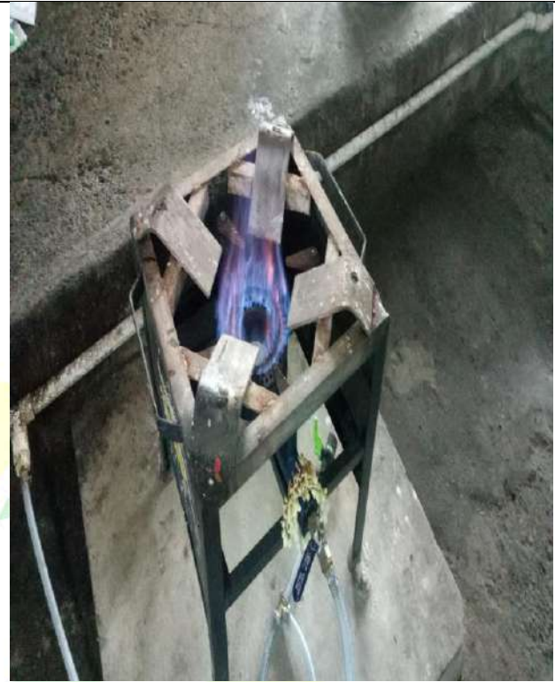
Figure 73: Burner Lit by Biogas
