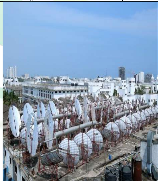
Figure 26: Solar cells on roof top
