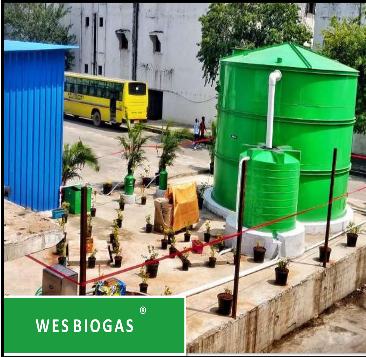
Figure 67: 1Ton/day Biogas plant Installed and Commissioned at Sathyabama Institute of Science and Technology, Chennai
