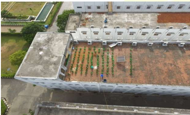
Figure 15: Roof top Solar Panel
