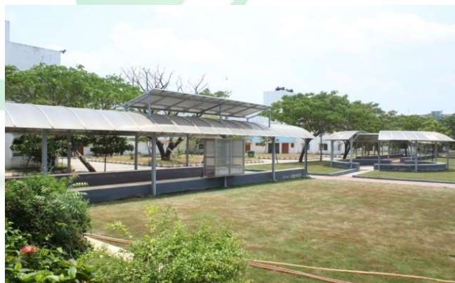
Figure 18: Solar panels with controller
