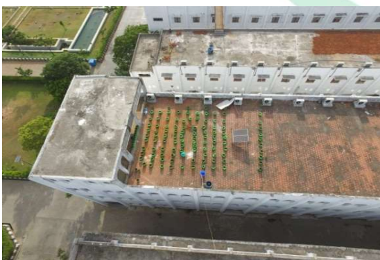
Figure 48: Roof top solar panel
